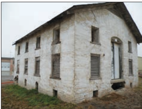
Historic structure at 63d facility in Laredo, TX
