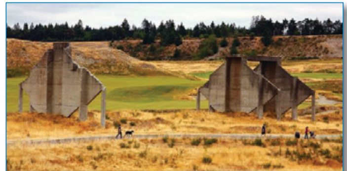
Remnants of the gravel bins, with walking trail in front and the 18th fairway in the background (photo by Amanda McLean)
