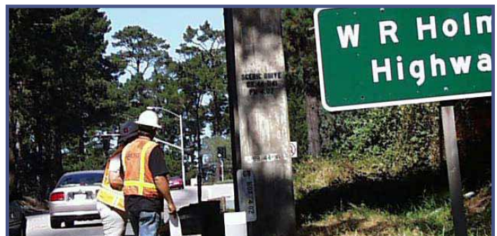
Route 68 (Holman Highway) Field Investigations.
